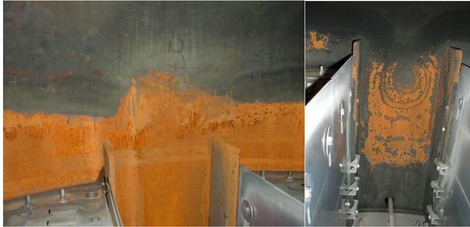
**Figure 8** Contactor Wall Corrosion in Tray Liquid holdup Area and Downcomer
